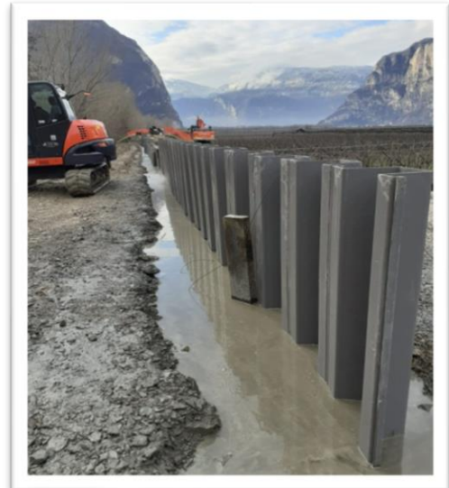
Rome (Italie) – 11000 m 2 – sealing wall (cut-off wall)
